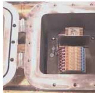
GAUGE POWER SUPPLY WITH ZENER BARRIERS
